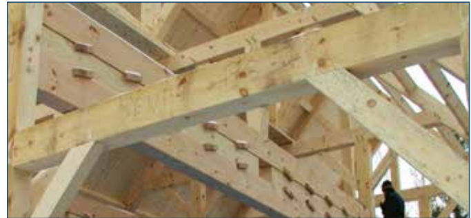
Shown here is a tri-laminate keyed beam that has a designed gap in the center lamina.
