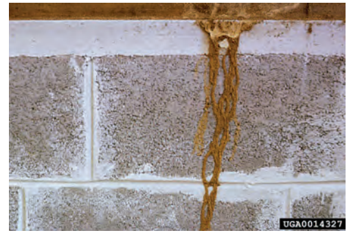
Fig. 27 Shelter tubes on concrete block surface, built by subterranean termites Reticulitermes Holmgren to communicate with ground, shown in Gulfport, Miss.
